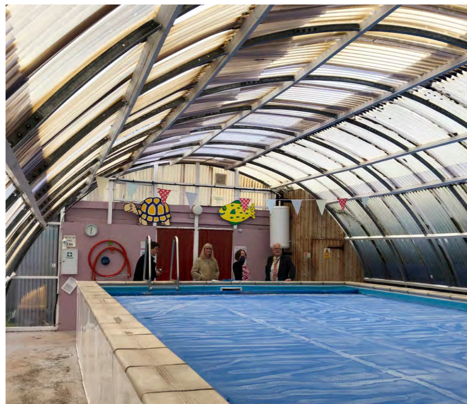
Interior of Swimming Pool Polytunnel roof
