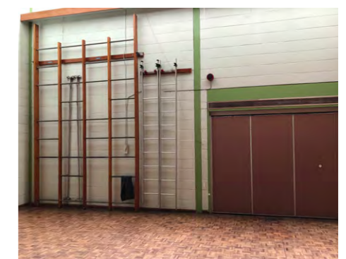
Hall PE Equipment with doors to table store
