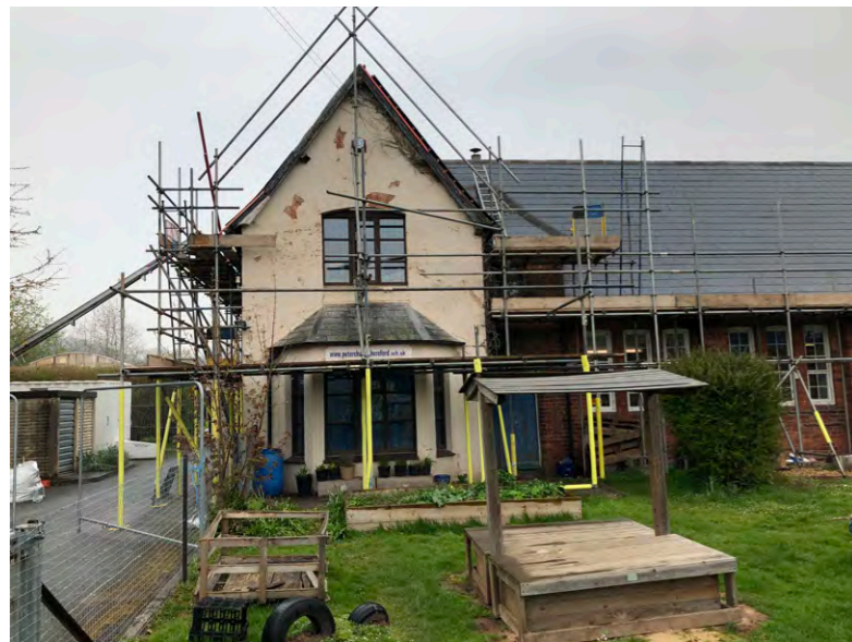
1. Original school building facing the front of the site
